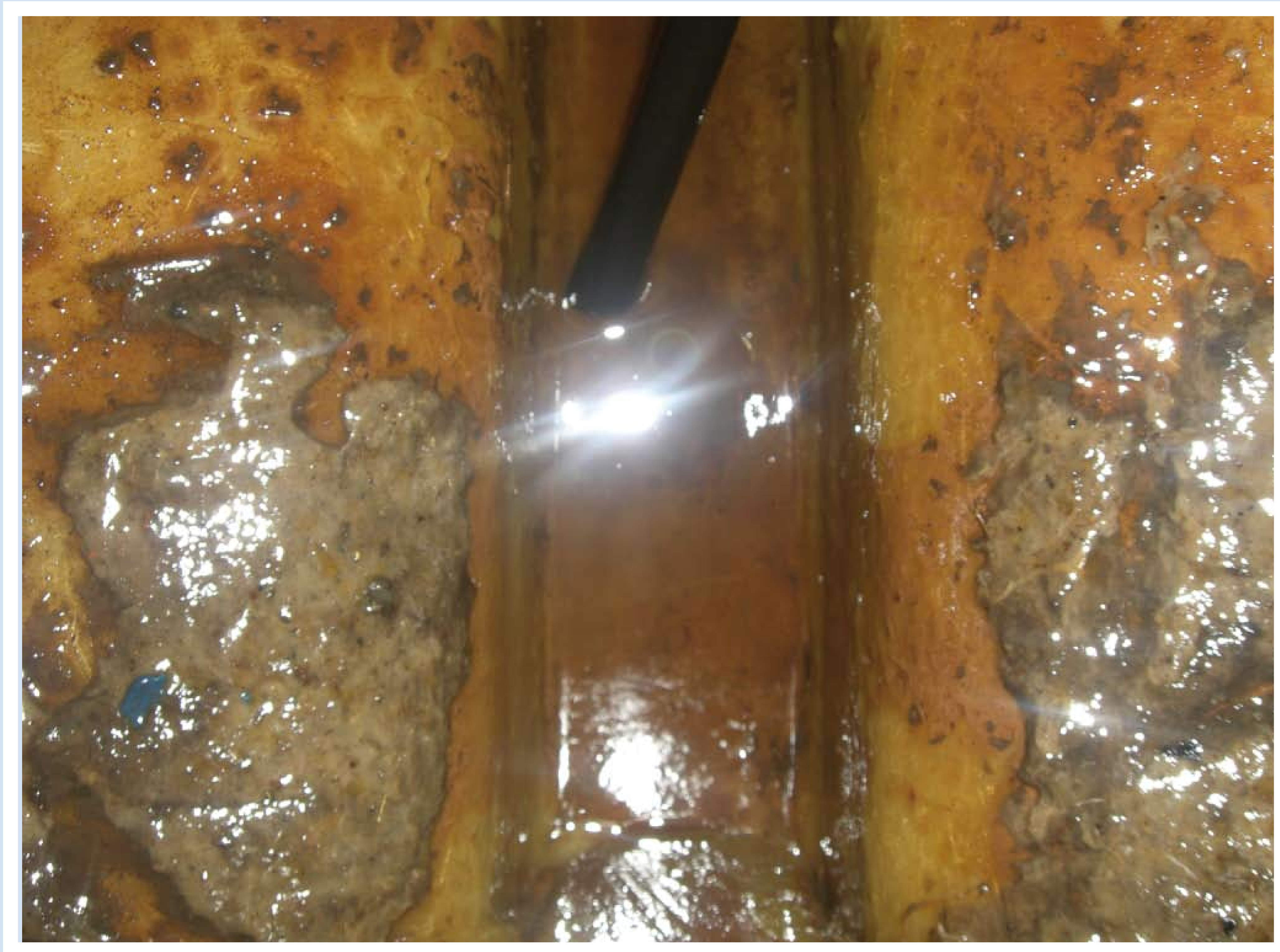
biofilm on a tank wall
